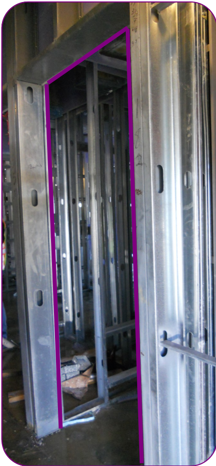
Fig 1. Rough opening for hollow metal frame
