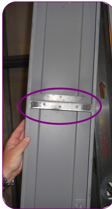
Fig 2. Clip detail added to hollow metal frame
